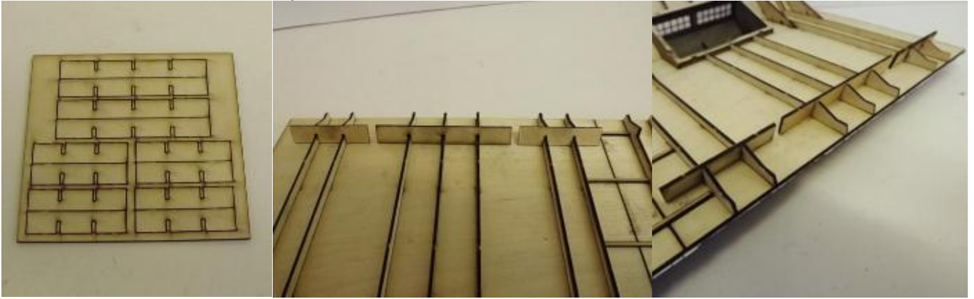
PHOTO 11D: Glue soffit boards in place.
